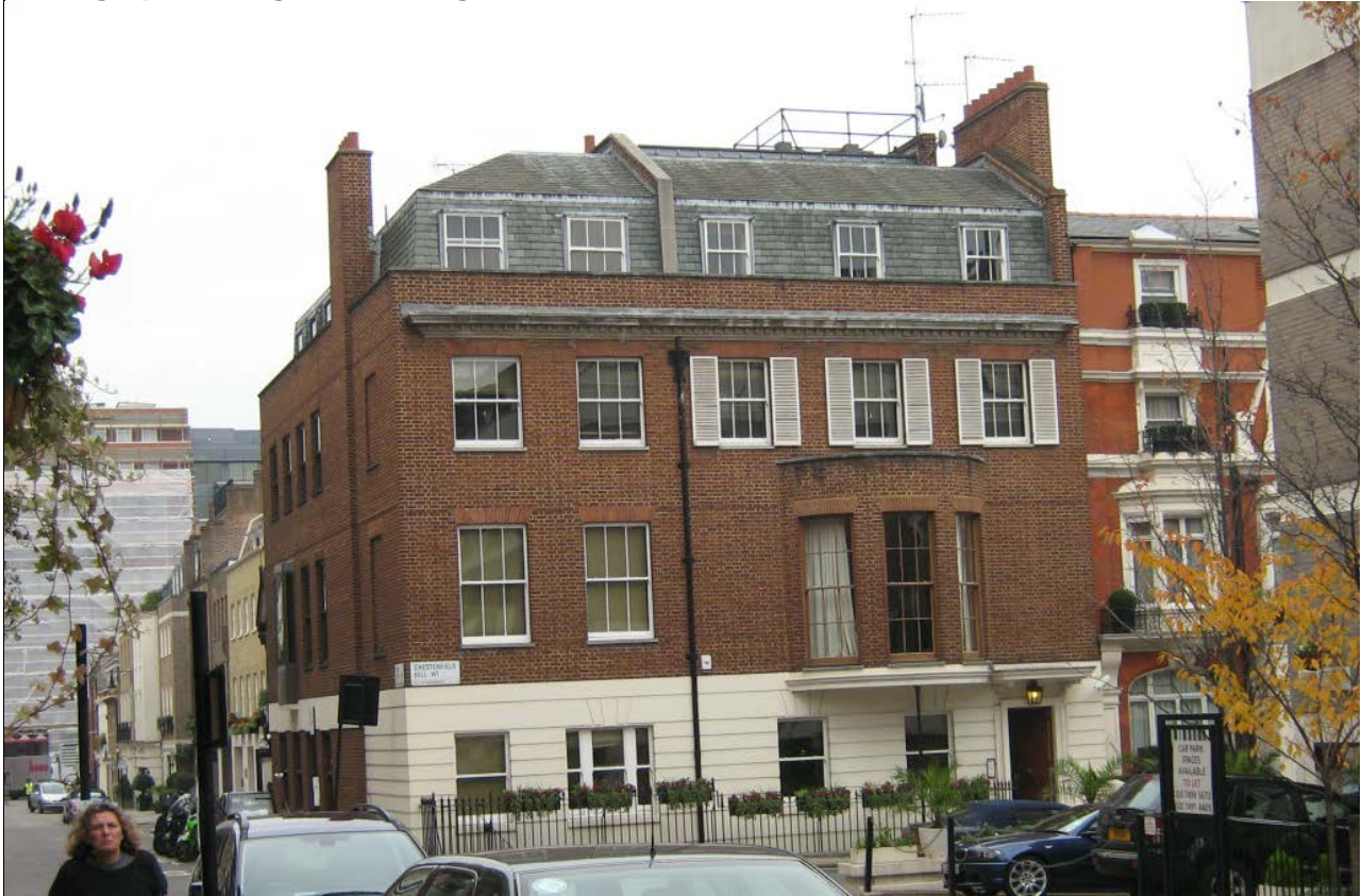
Photograph 1: Original building before demolition
